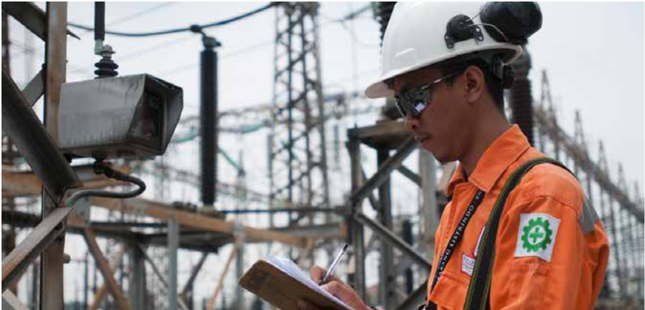
▲ Switchyard di PLTGU Jababeka Switchyard at GSPP Jababeka
