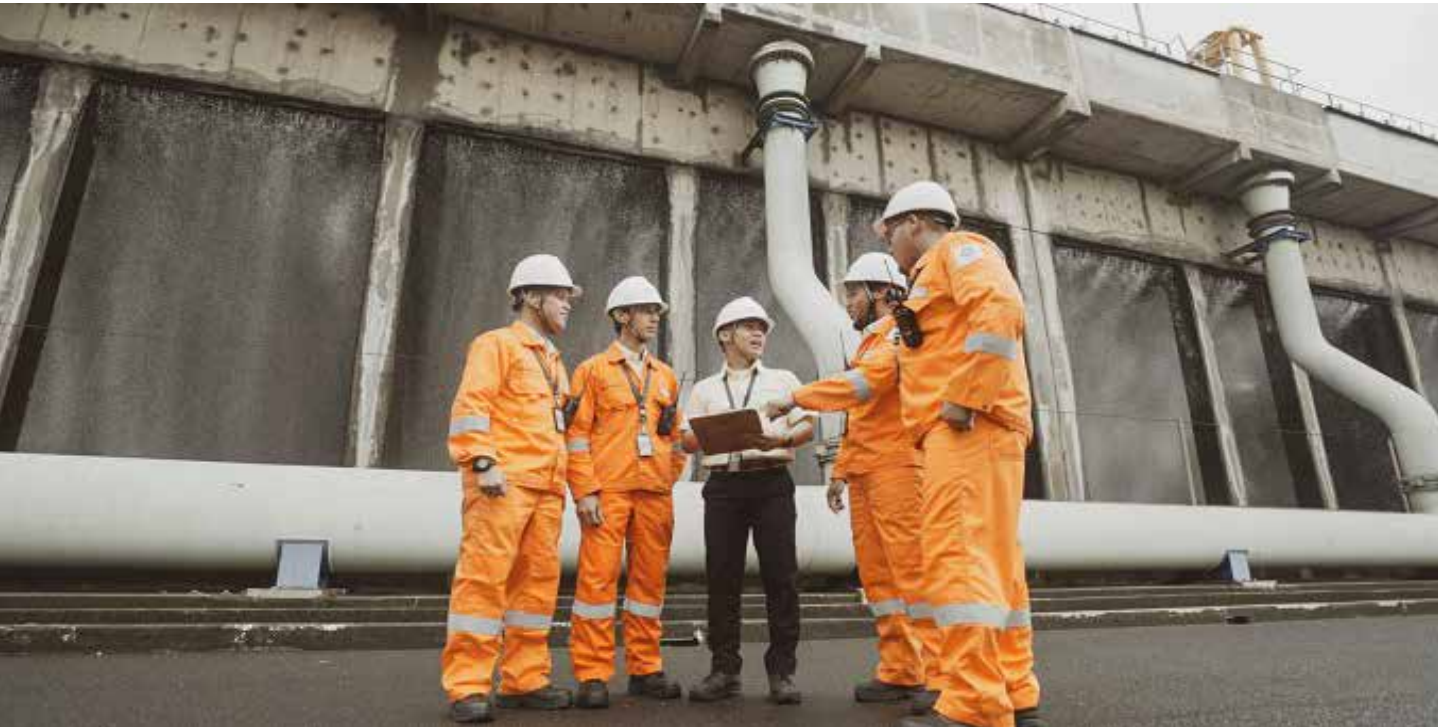
▲ Cooling Tower di PLTGU Jababeka Cooling Tower at GSPG Jababeka
