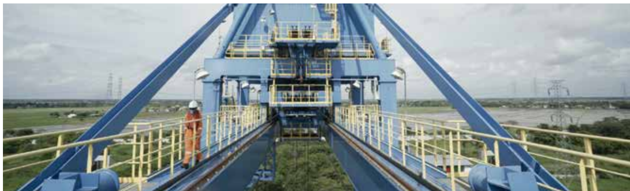
▲ Fasilitas Coal Handling di PLTU Babelan Coal Handling Facility in CFPP Babelan
