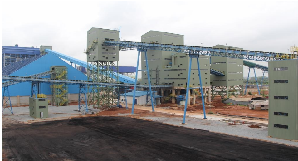
Transfer Tower and Belt Conveyor
