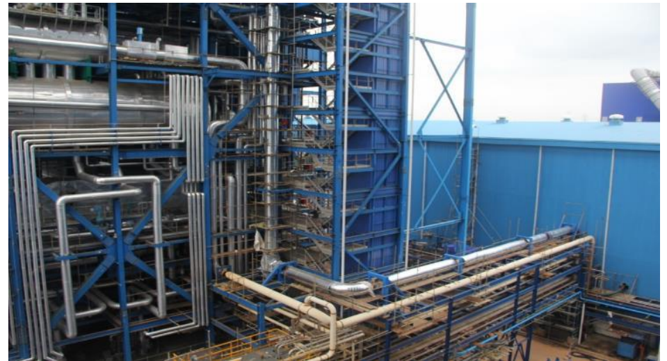
Boiler 2 and Pipe Bridge to STG
