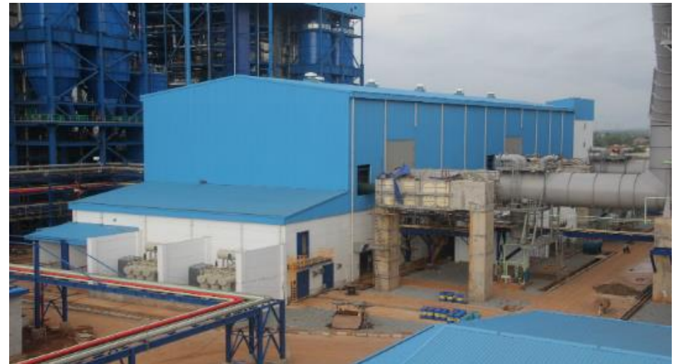
Steam Turbine Hall
