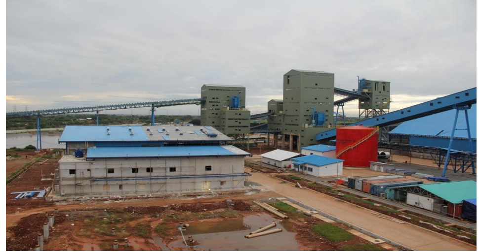
Office, Workshop, Warehouse Construction on Progress
