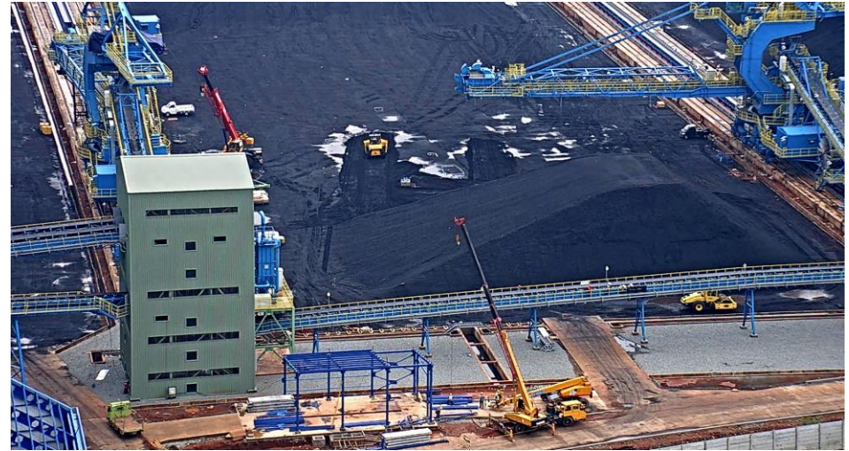
Stock pile and Transfer Tower
